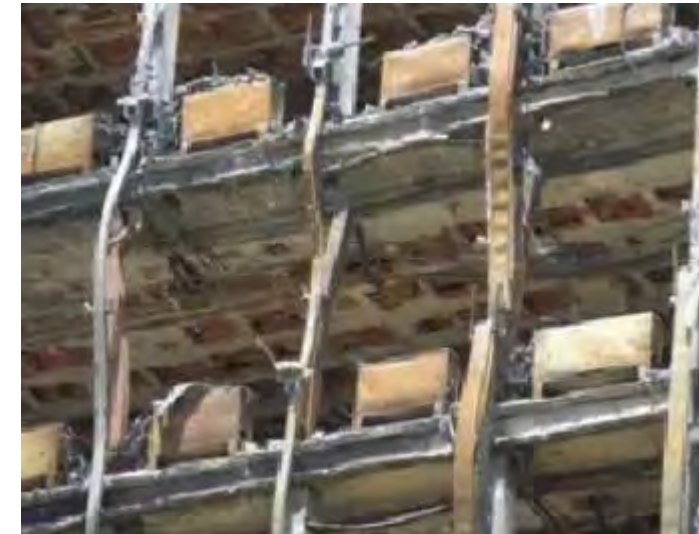
Buckling at floor 9
